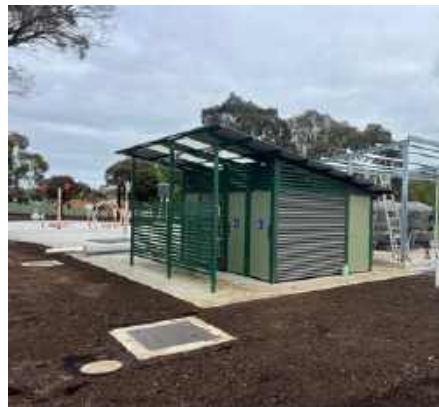
Splash Park Facilities. Image supplied by the City of Ballarat
